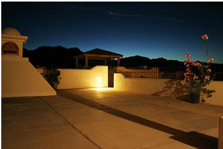
Many of the village homes in Loreto Bay feature rooftop terraces. Photo by Simmons Buntin.
