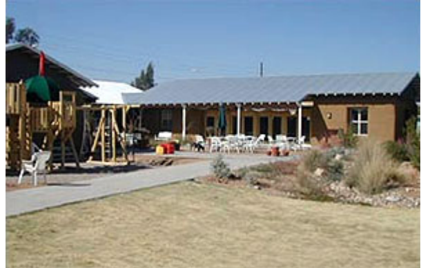
Sonora's strawbale common house features wide, deep porches and plenty of community gathering areas. Photo courtesy Sonora Cohousing.
