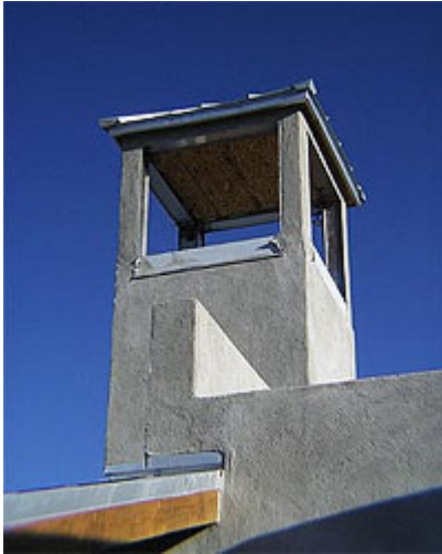
North face of the 30-foot cool tower, recently stuccoed. Photo by Wilson Graham.
