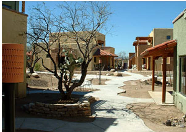
Phase 2 residences at Stone Curves, including salvaged mesquite and prickly pear. Photo by Simmons Buntin.
