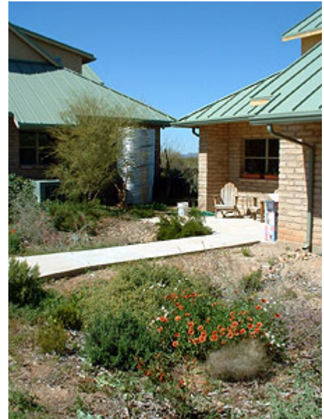
Milagro water harvesting features include cisterns and swales. Photo by Simmons Buntin.
