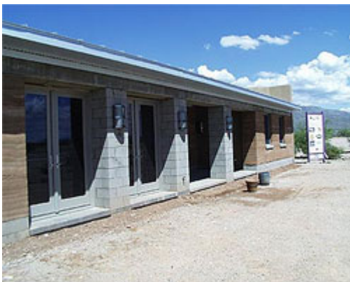
South side of residence with completed facade, CMU pillars, and rammed-earth walls. Photo by Wilson Graham.
