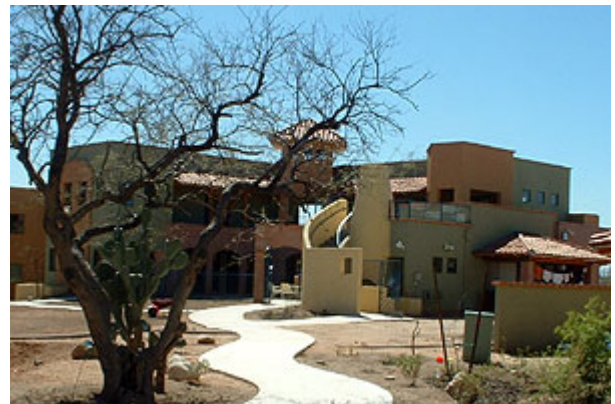
The Stone Curves common house is the largest in the Tucson area. Photo by Simmons Buntin.
