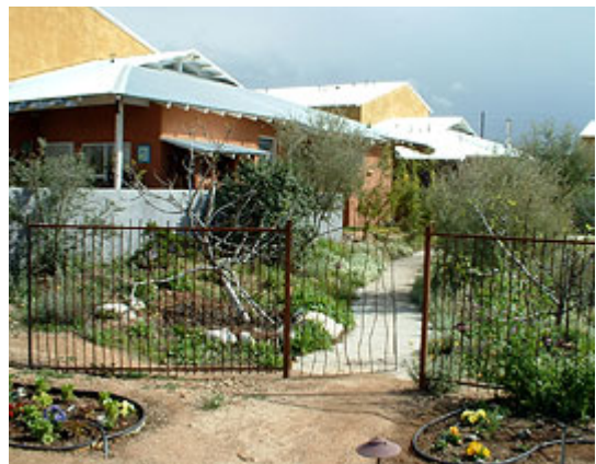
View from the community garden, with its custom rebar fence and gate. Photo by Simmons Buntin.
