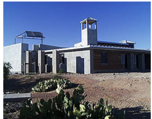
View from southwest following stucco and solar water heating system completion. Photo by Wilson Graham.
