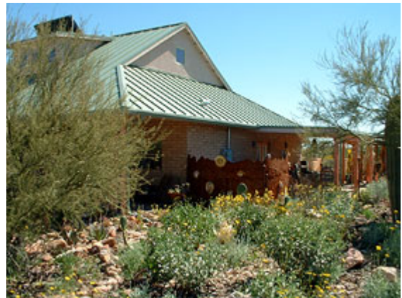
As at Milagro, environmental preservation and resource efficiency are critical for all of Tucson's cohousing developments. Photo by Simmons Buntin.
