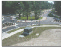
Roundabouts make drivers slow down as they approach an intersection, and separate the movements of people and vehicles to reduce conflicts and increase safety.
